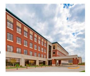
The building consists of structural concrete frame with brick and stone masonry veneers, curtain wall and punch windows. Site improvements include new utilities, concrete and asphalt paving, sidewalks and plazas.
